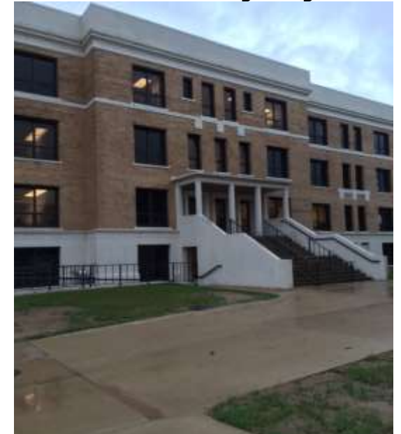
Milner Hall – North Entrance from Northside Parking Garage
